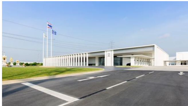
Entrance to the engine plant at Mazda Powertrain Manufacturing (Thailand)
