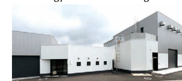
Material MBR Building / Data-Driven Technology Research Building
